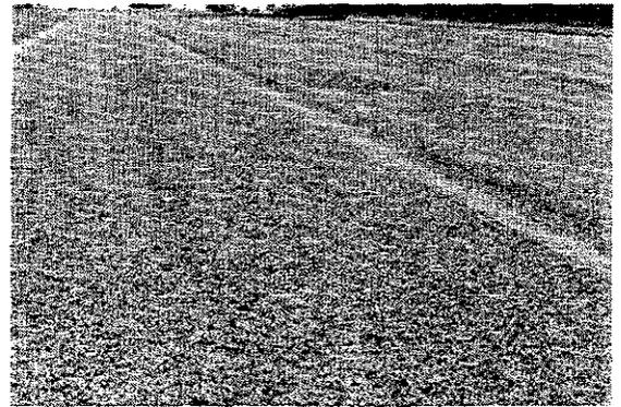
Photograph #10: Asphalt with Excess Tar.
