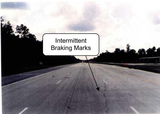
Figure 5. CS2 – Tire Marks (Direction of Travel View)
