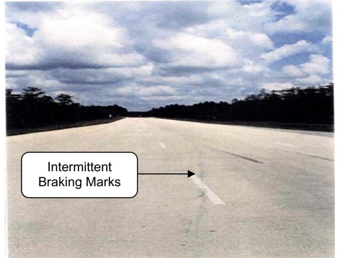
Figure 6. CS2 – Tire Marks (Opposite Direction of Travel View)
